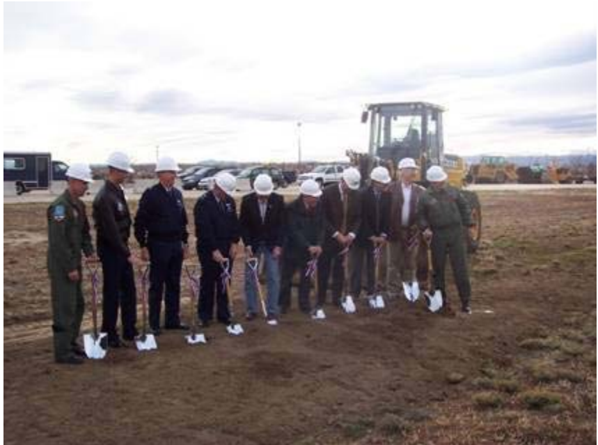
The group preparing to break ground for the new construction at Buckley AFB.
